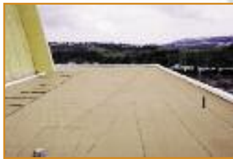
GSA Chet Holifield Federal Building Laguna Niguel - California, 2004
